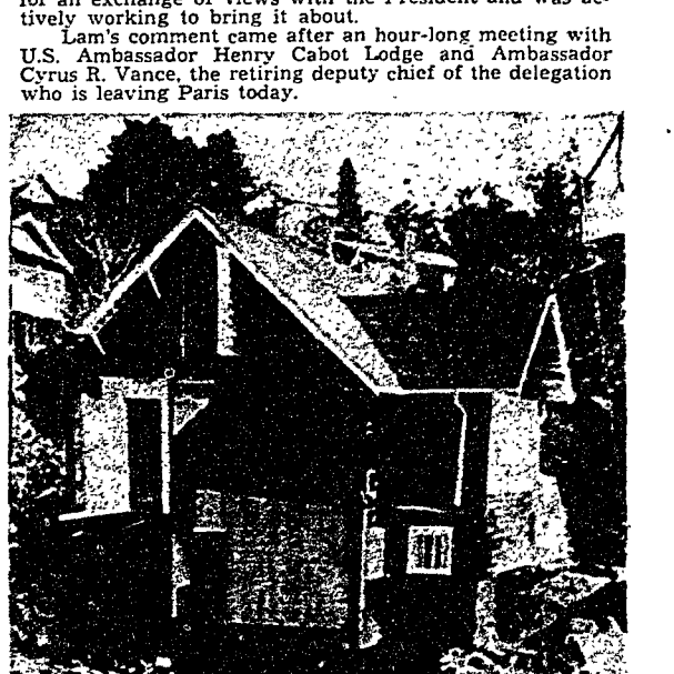
A HILLSIDE HOME in the Mt. Washington area of Los Angeles has already lost its playground and bathroom — the victims of earthshakes resulting from recent rainstorms. A city official said the worst slides may be yet to come.
